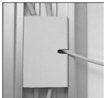
**8.2** Press one side of the Cover into channel, routing cables behind Cover and through notches. Squeeze Cover and insert other side into channel.
