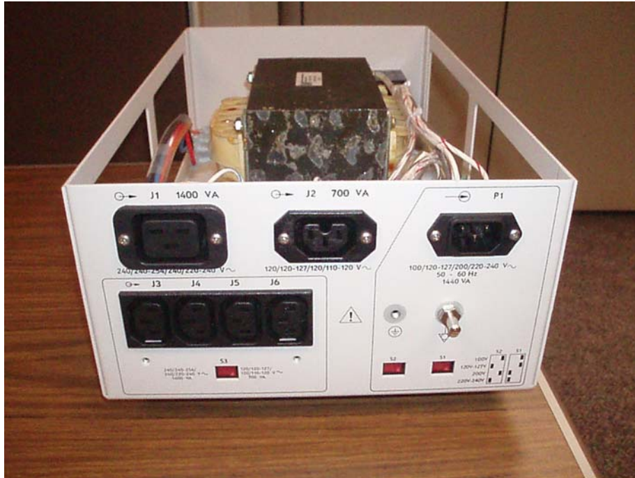
Figure 1 (picture of unit with cover off – removed with Phillips Screwdriver)
