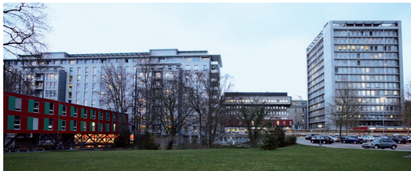
Regional Hospital Winterthur, Switzerland
