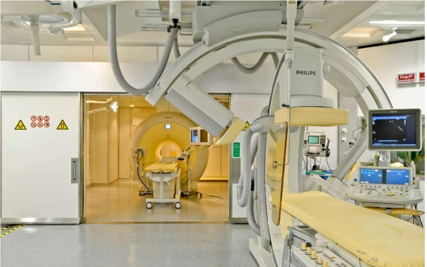
The hybrid system: a Philips Achieva 1.5 Tesla Cardiac MR, Philips Allura Xper FD 20/10 biplane X-ray and Philips iE33 echocardiography system with a 3D TEE probe all in one room
