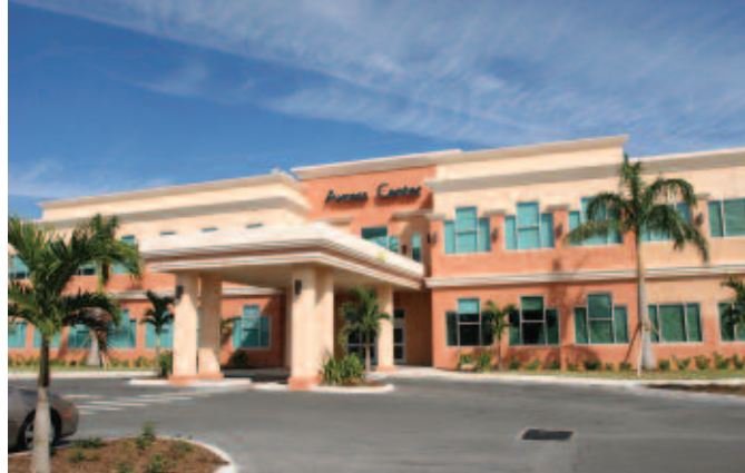
Access Diagnostics Imaging Center, Sarasota, Florida, USA
