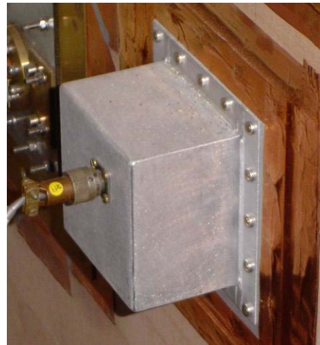
Figure 7 7T coldhead power filter.
