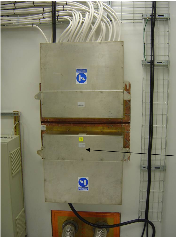
Figure 2 7T Shim filter assembly (lower unit) RF feedthrough.
